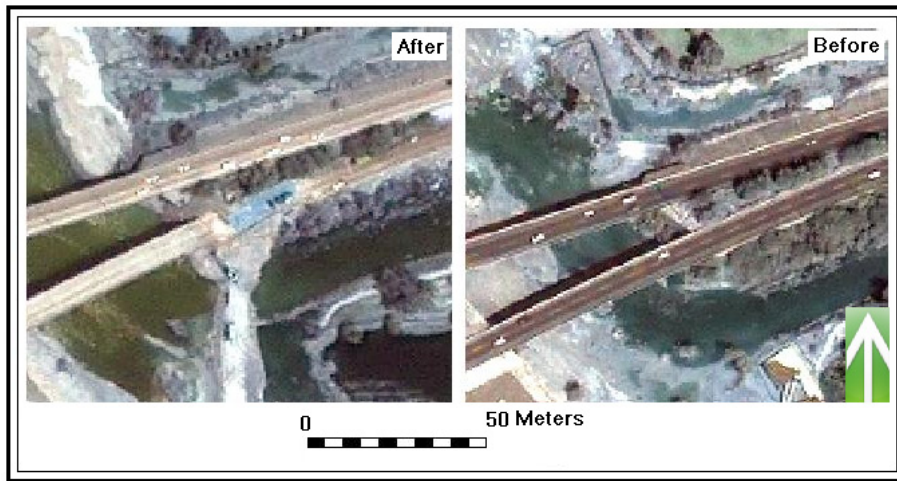
Figure (6) a damaged part of a bridge on Alqurm area Bridge (left), the bridge before the cyclone (right)
